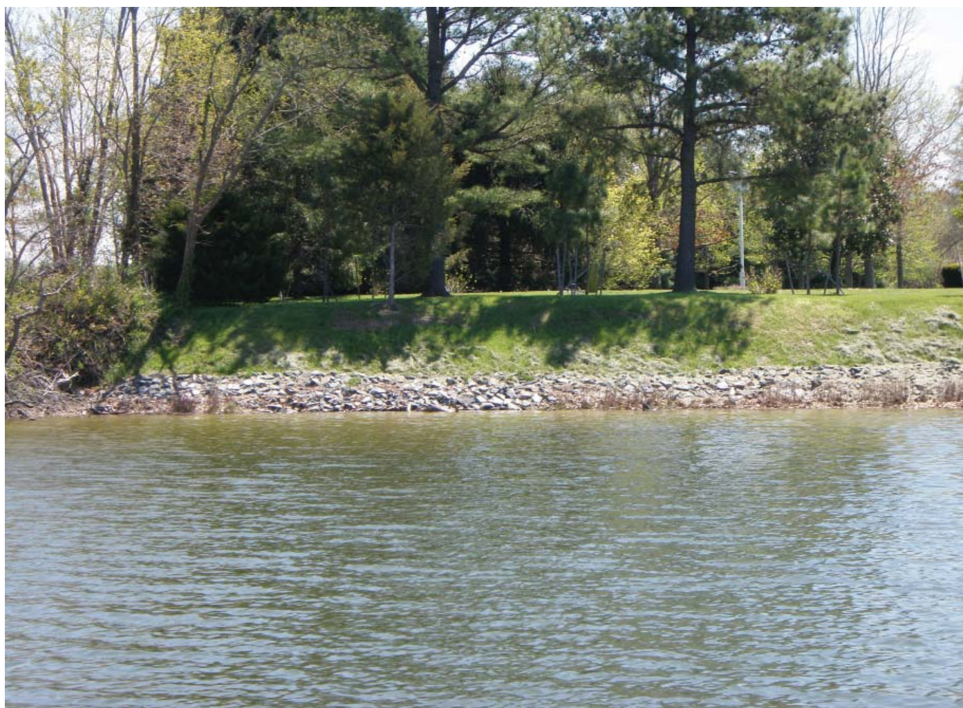
Riprap along the Tred Avon. Photo credit: NOAA National Centers for Coastal Ocean Science
